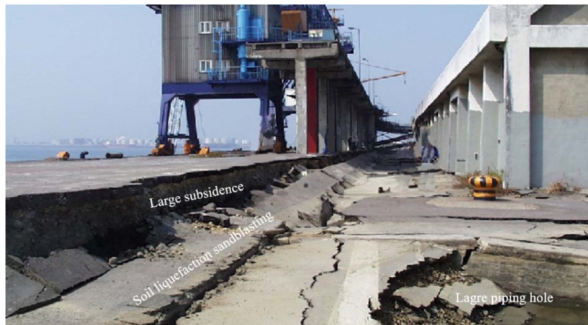
Figure 2. Damage to the rear-line region of the dock caisson induced by the 1999 Jiji earthquake, Taichung Port (Lai et al., 2007).
